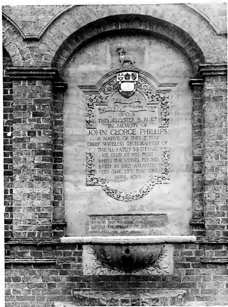
FIG. 203.—TABLET SET IN WALL OF THE JOHN GEORGE PHILLIPS MEMORIAL, GODALMING.
